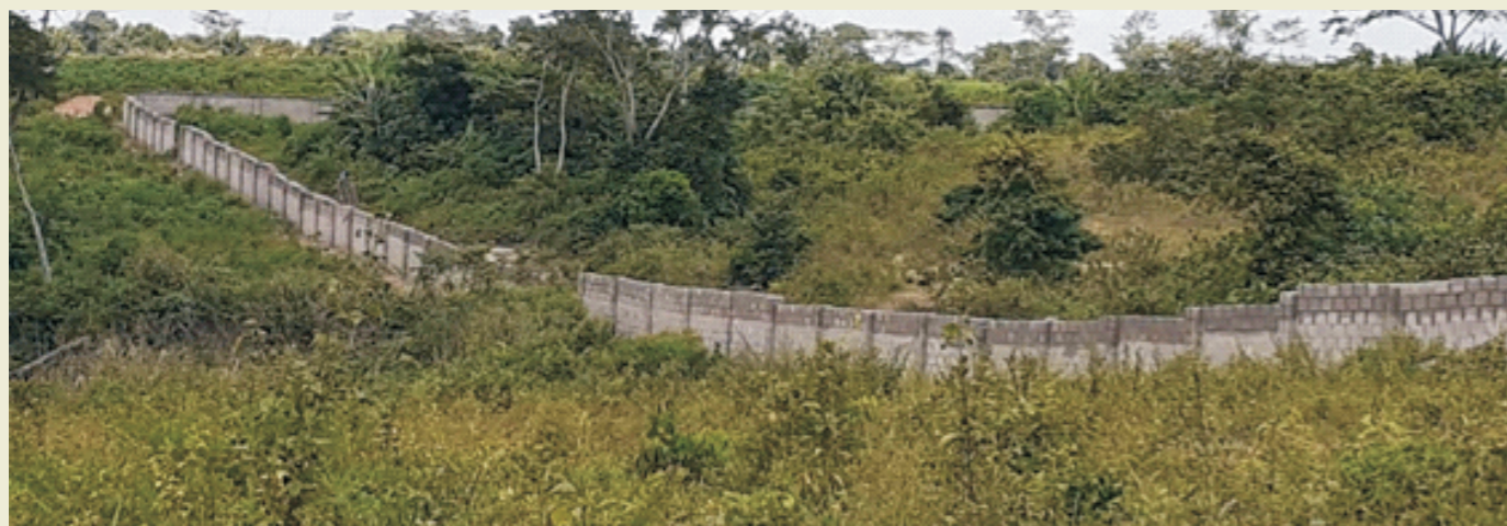
COMPLETED SECTIONS OF THE FENCE
