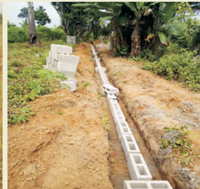
FABRICATION OF BLOCKS, EXCAVATION AND FOUNDATION WORK
